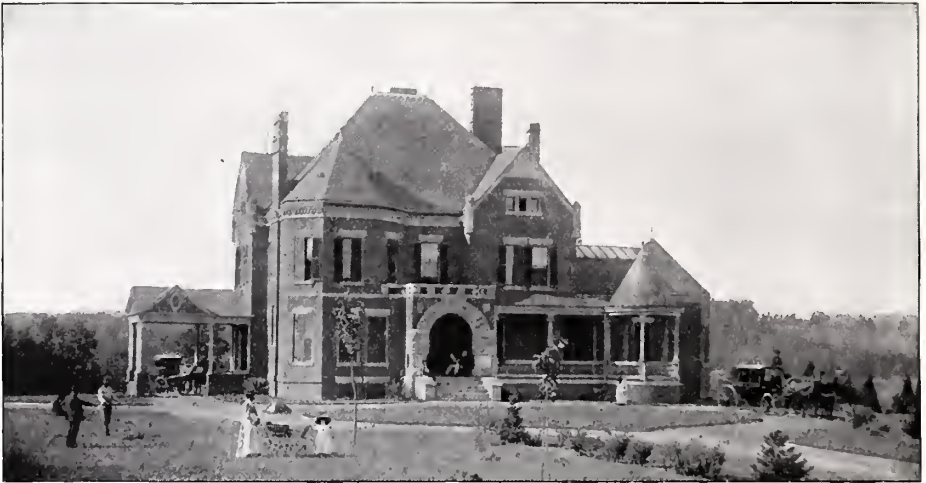
RESIDENCE OF J. E. LUTZ, MERCHANT, KNOXVILLE, TENN. Baumaunn Bros., Knoxville, Architects.
